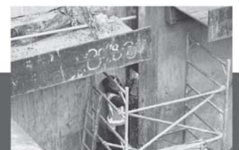
Onsite welding in New Lynn Railway trench.
